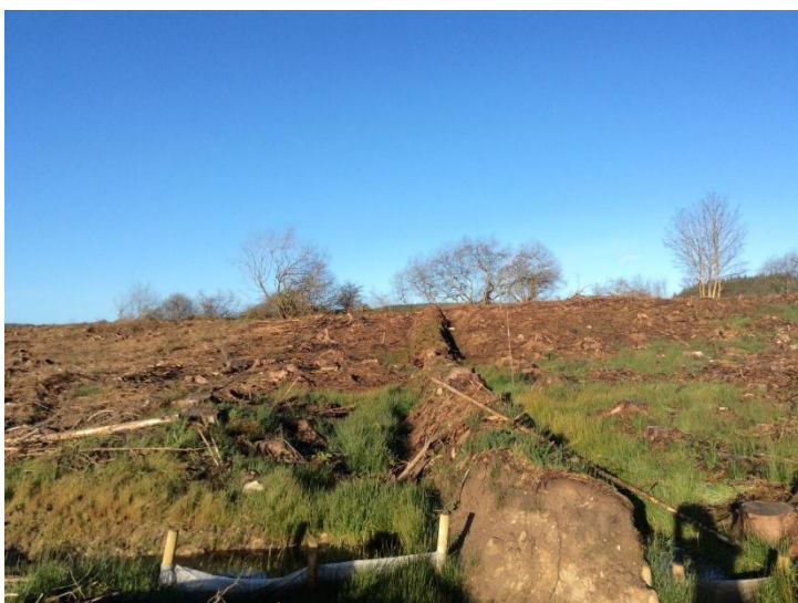
Plate 24: Proposed road to T8 through clear-felled forestry, looking NW.
