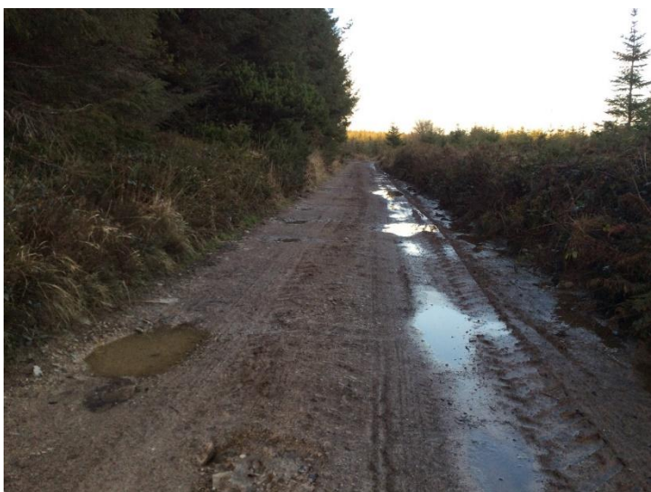
Plate 45: Existing road due for upgrade between T20 and T21, looking NE.
