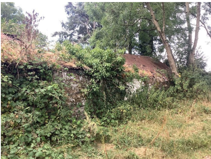
Plate 66: Ruinous structure CH4, looking NW.
