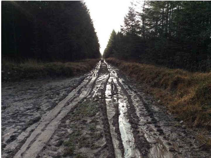
Plate 7: Existing track due for upgrade south of T2, looking SSW.
