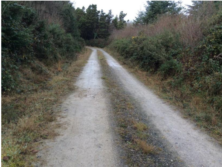
Plate 16: Existing road due for upgrade NW of T6.
