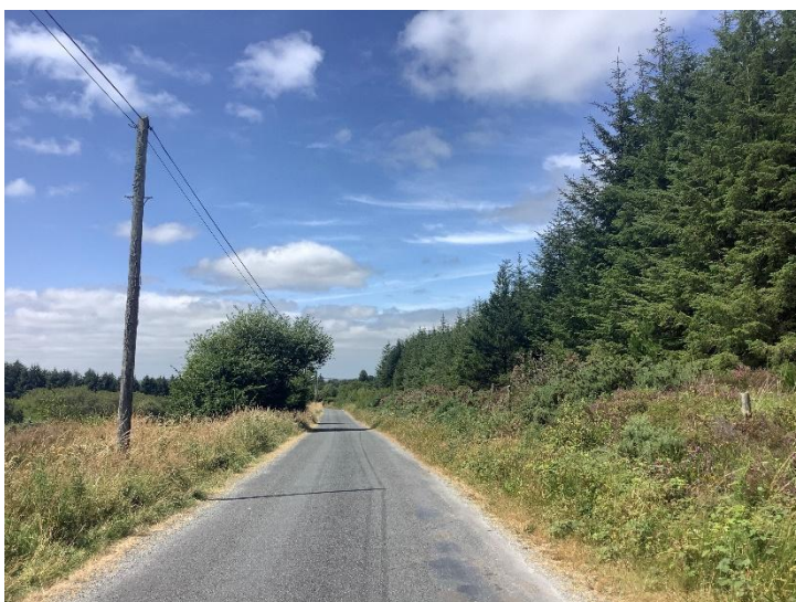
Plate 57: Proposed 110kV Underground Cabling Route further to west, looking WNW.
